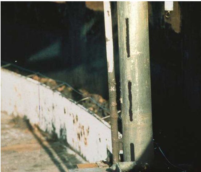
The Low Loss Mode enables full accuracy also in old and worn still-pipes.
